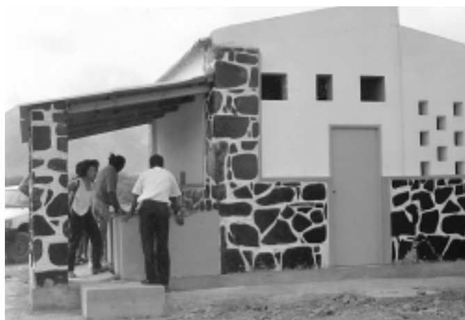
Typical water distribution point that includes washing stands and showers.
