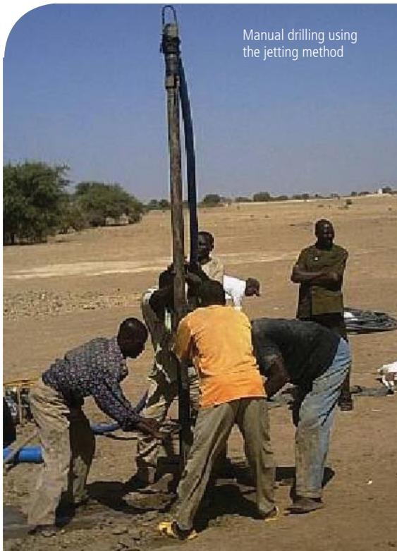
Manual drilling using the jetting method
