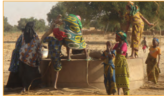
Concrete lined dug-well
