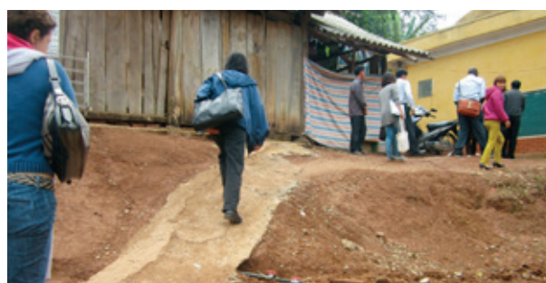
Photo 3: Footpath leading to school manager's office at a pre-primary school in a rural community
