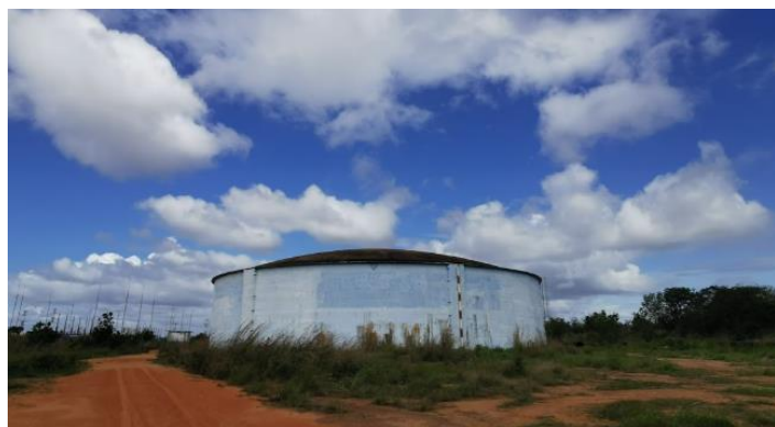
© UNICEF/2021/Simon. 20,000 m 3 water tank, capable of distributing chlorinated water to more than 250,000 people thanks to UNICEF support.
