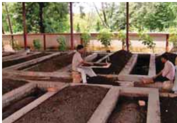
Overground brick lined compost pit
