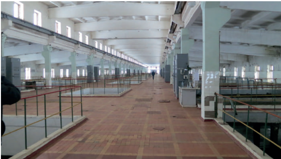
Verkhniokalmiuska WTP filter hall
