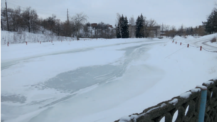
SDD channel with ice cover at the intake for the Pumping Station 3
