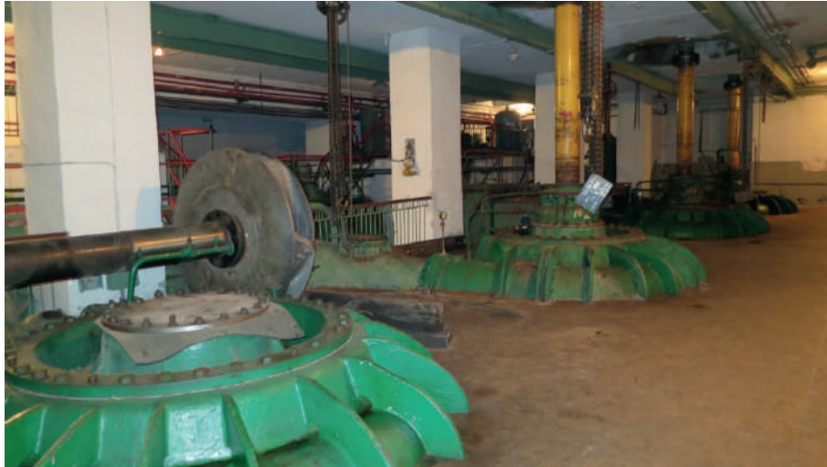
The pumps of Pumping Station 3, No. 1, dismantled
