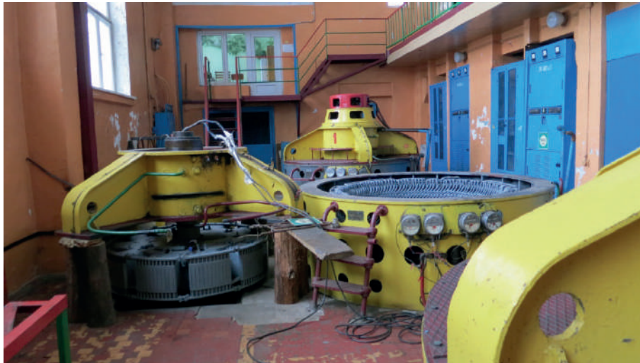
Machine hall of 4 th Lift Station, unit no. 2, dismantled motor
