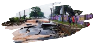
Rádio Renascença/Flood damage after heavy rains, Timor-Leste/ 2021
