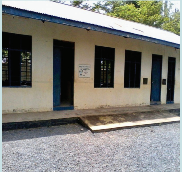
A building for the special unit at a primary school in Geita Town Council, built with funds from Plan International. Classes are, however, inadequate for the unit
