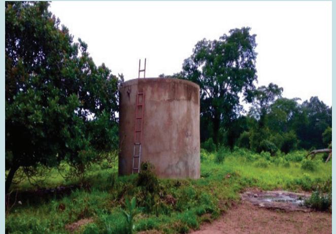
Water tank constructed with TASAF funds in one of the secondary schools in Lindi DC
