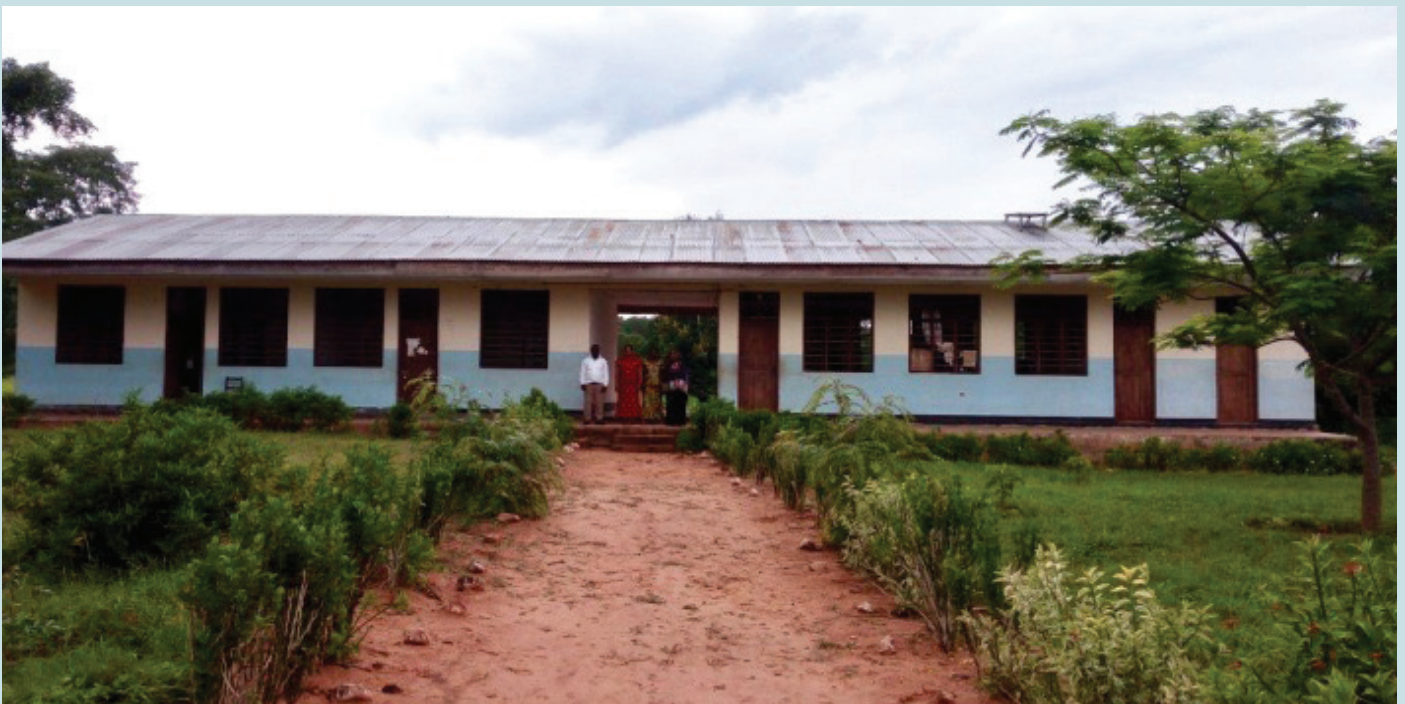
Administration block built with TASAF funds in one of the secondary schools in Lindi DC
