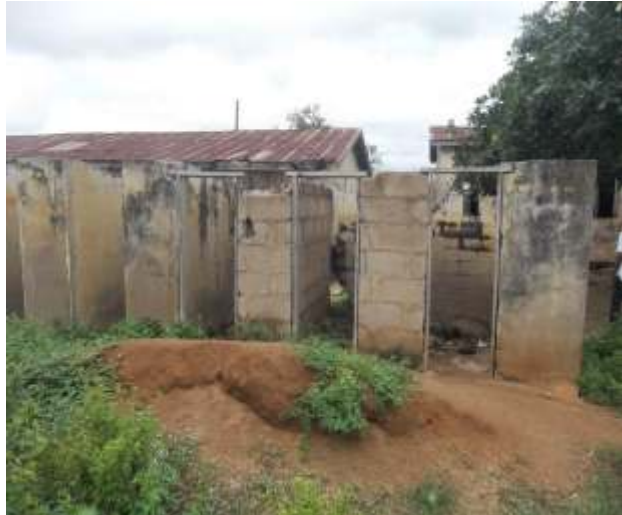
Toilet compartment without roof & doors. Credit: Tomi Ogunsanwo 2015
