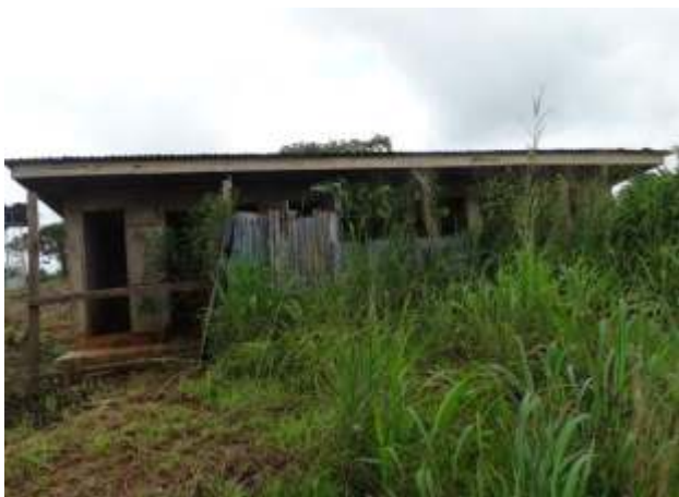
Rural school toilet overgrown with bush. Credit: Nkadi Onyegegbu
