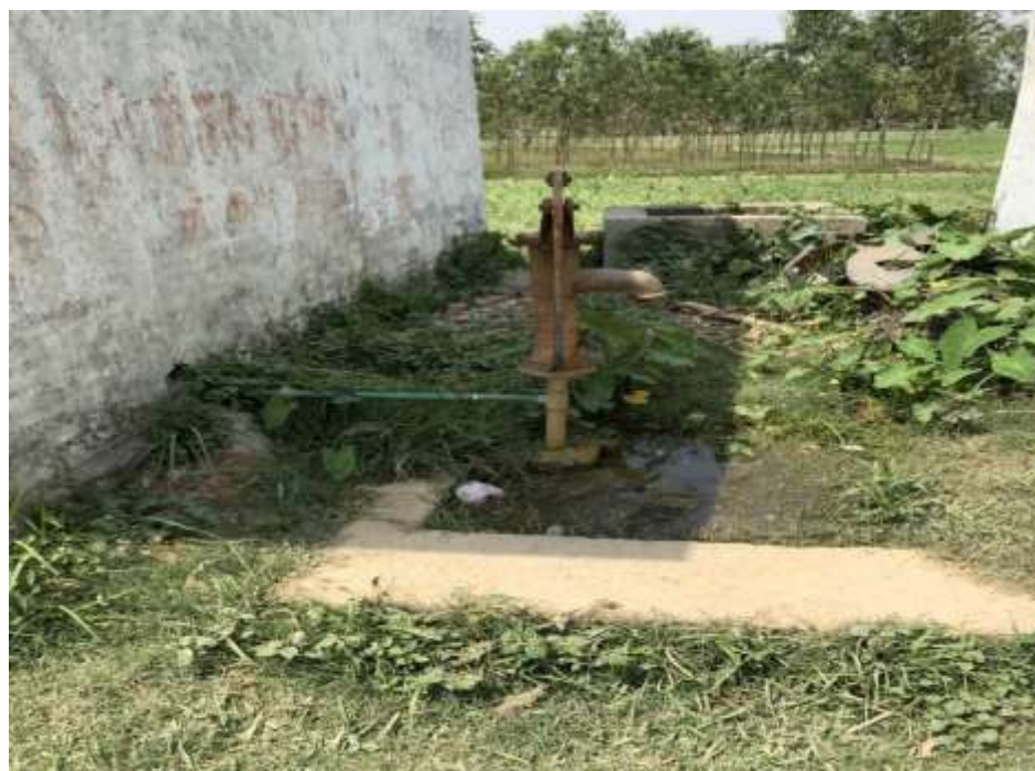
Figure 8 Tubewell as main water source in School
