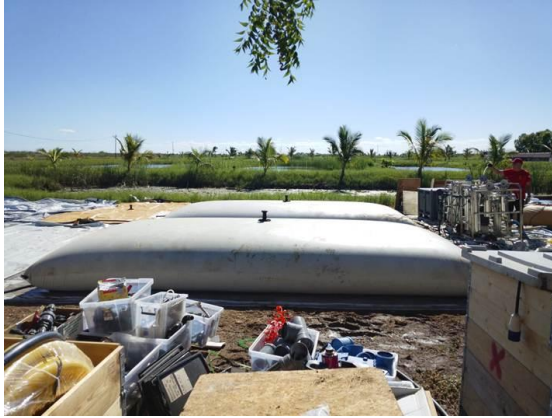
Portable water treatment unit by the Spanish cooperation which is producing an average of 30 cubic metres of water to support Hokwe accommodation centre and host communities-Chokwe district
