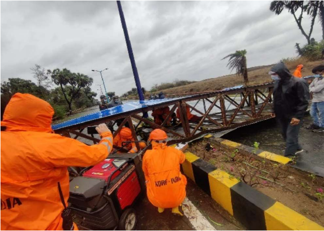
NDRF personnel carrying out road clearance work-Diu
