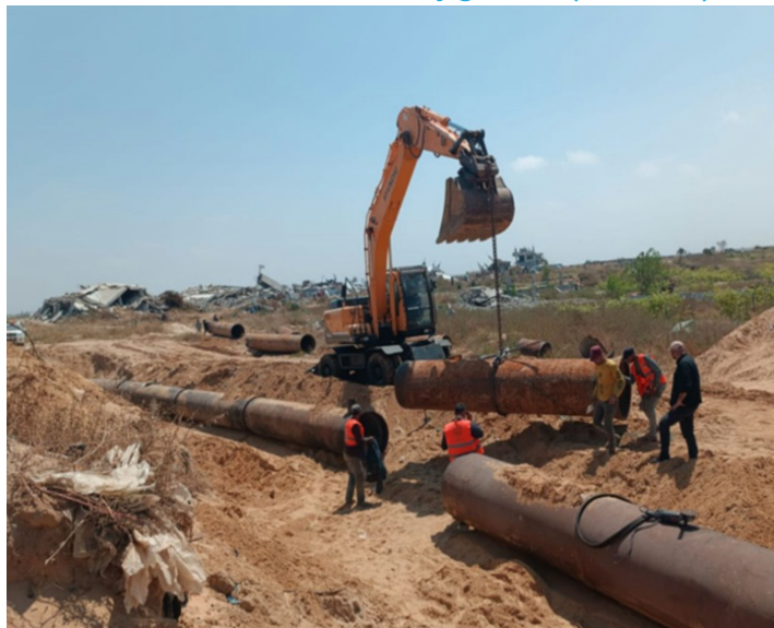
Maintenance of the wastewater trunk line in the south of Gaza City.
