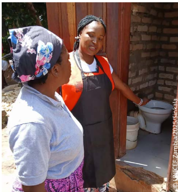
Agness collects data and inspects a household toilet to assess safely managed sanitation, supporting accurate reporting and better hygiene practices in Zambia.
