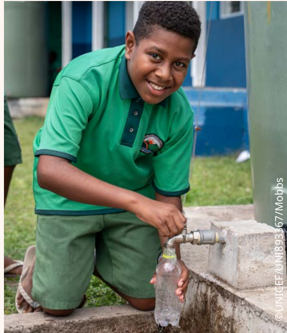
A student fills his bottle from a water tank installed by UNICEF at earthquake-affected Suango School, Shefa Province, Vanuatu in October 2025.
