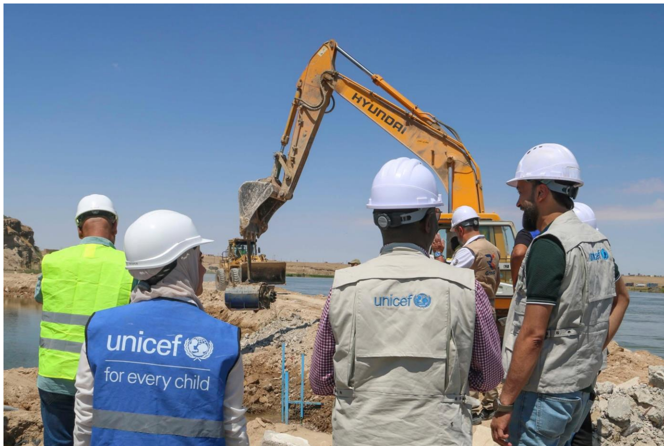
Engineers are working to protect the embankment of the Euphrates River so that the critical structure of the Al Baghouz Water Treatment Plant in Deir-ez-Zor Governorate is not flooded. @UNICEF/Syria-2026/Bashar Al Kheder
