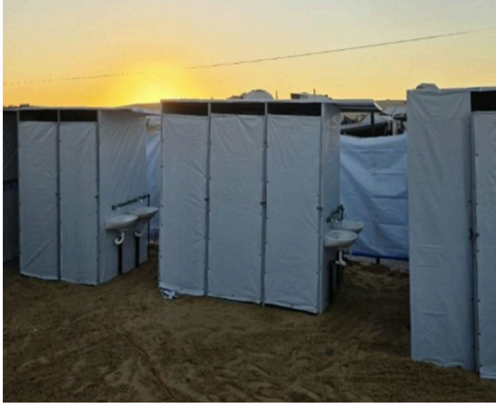
UNICEF provides water and sanitation services in Learning Centres and Health Care Facilities in the Gaza Strip.
