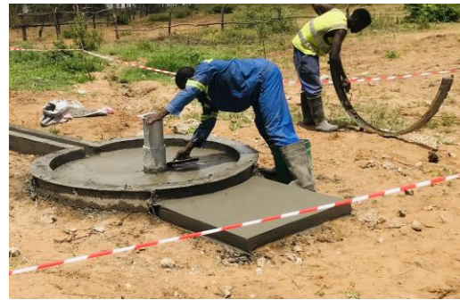
Borehole rehabilitation ongoing in Sitoti RHC in Sioma district. Credit: UNICEF Zambia/2024/Musa.
