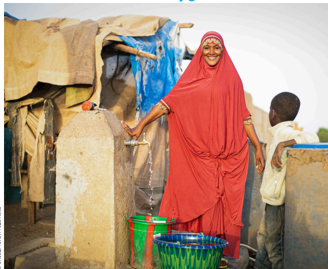
UNICEF and its partners rehabilitated and equipped an old borehole into a simplified water supply system. This emergency project installed 3 water fountains to provide a access to safe drinking water
