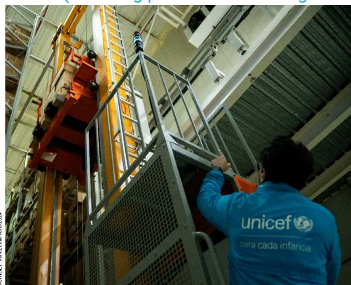
Hugo Bravo, UNICEF Supply Officer, supervises the delivery of Venezuela's largest robotic warehouse, rehabilitated by UNICEF to increase cold chain capacity and vaccine storage. May 2024
