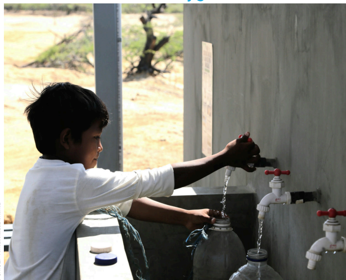
Boy accessing water in the Wasulee community battery, built by UNICEF. The battery works with a windmill and benefits more than 2,000 Wayúu indigenous people in Zulia state. April 2024.
