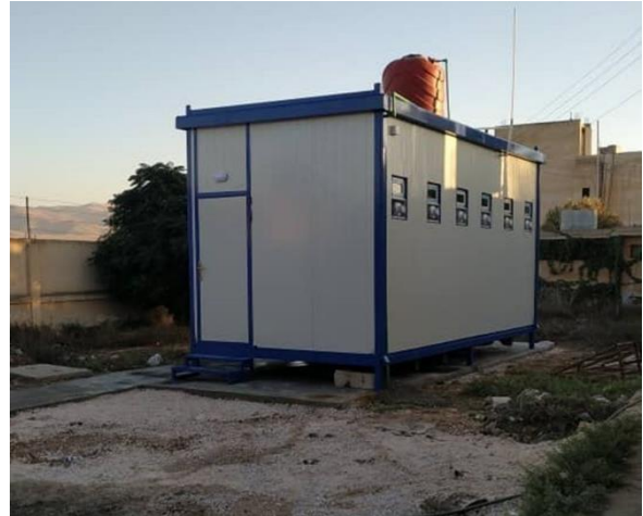
UNICEF-supported prefabricated toilet unit in Joussieh crossing point in Homs Governorate. © UNICEF/Rahman Khateeb
