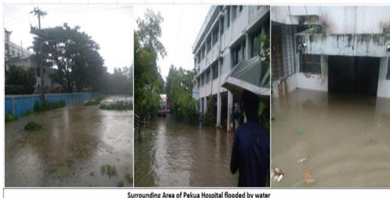
Surrounding Area of Pekua Hospital flooded by water
