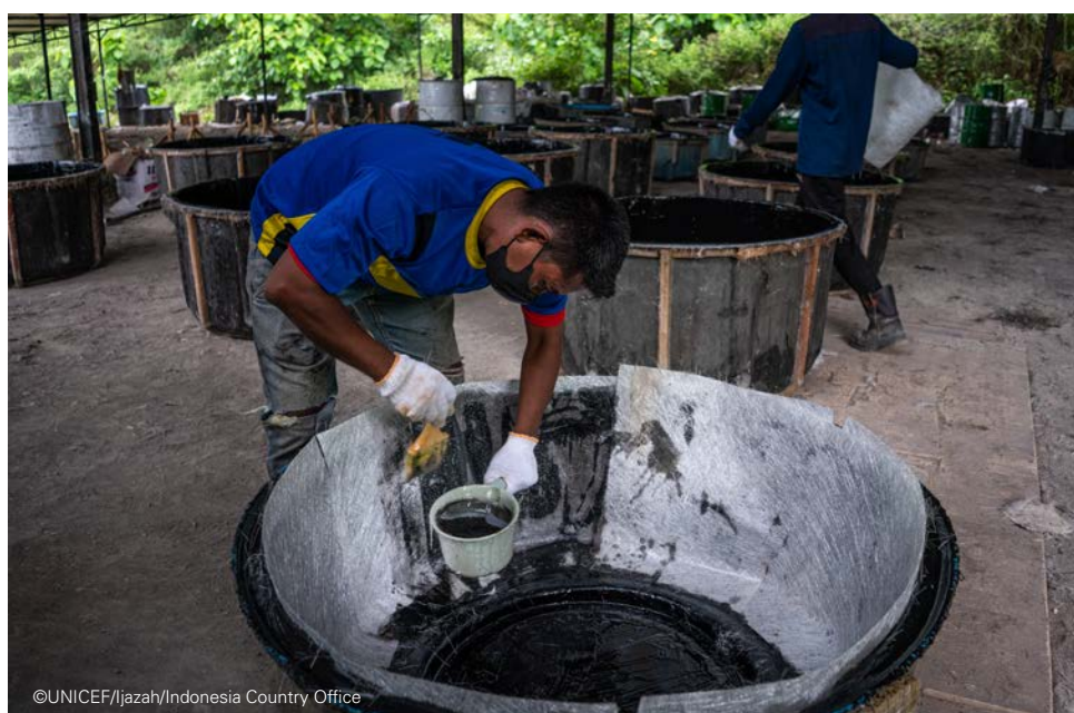
A local manufacturer builds a septic tank in Sumbawa Barat.
