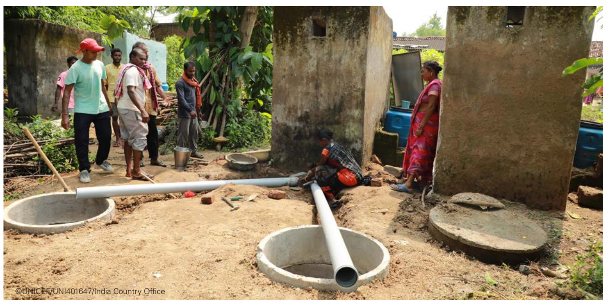
Toilets are being retrofitted in Odisha.
