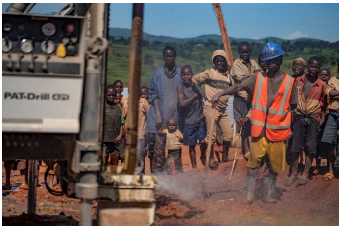
Onlookers cheer as a UNICEF drilling team hits water in the Rhoé camp for a new borehole. A new borehole at the Rhoé camps will increase water supply to 10 litres per person per day from 8 litres. UNICEF/DRC/2023/Mulala.
