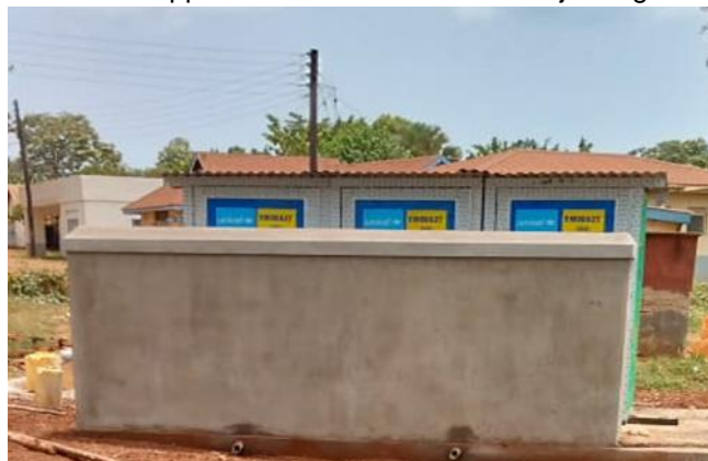
Figure 1: Mobile toilets installed at Jinja Regional Referral Hospital. Picture taken by Paul Kejira
