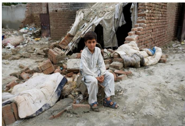
9-year-old Shafiq sits in the rubble of his home in Jalalabad, Nangarhar Province, eastern Afghanistan, which was destroyed during a flash flood that swept through the neighborhood on 15 August 2022.
