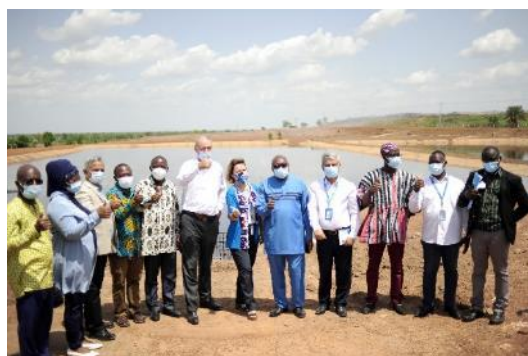
Netherlands Ambassador to Ghana, Officials from the Government of Ghana, and UNICEF Staff from Tamale Field Office and Accra launching the rehabilitated waste stabilization pond in Tamale, Ghana, 26 May 2021. ©UNICEF/UN339880/BUTA
