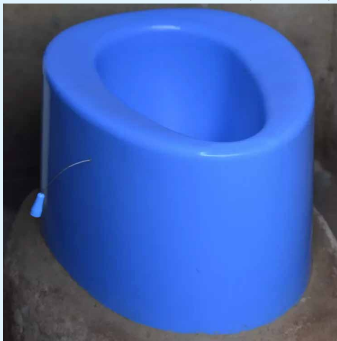
A sample SATO stool installed in a latrine
