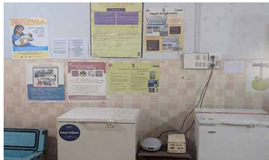
Figure 14: Cold Chain Room
