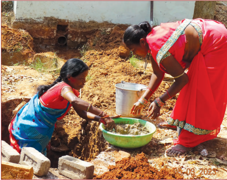
A woman mason independently constructing a twin-pit toilet in her house in Sambalpur, Odisha
