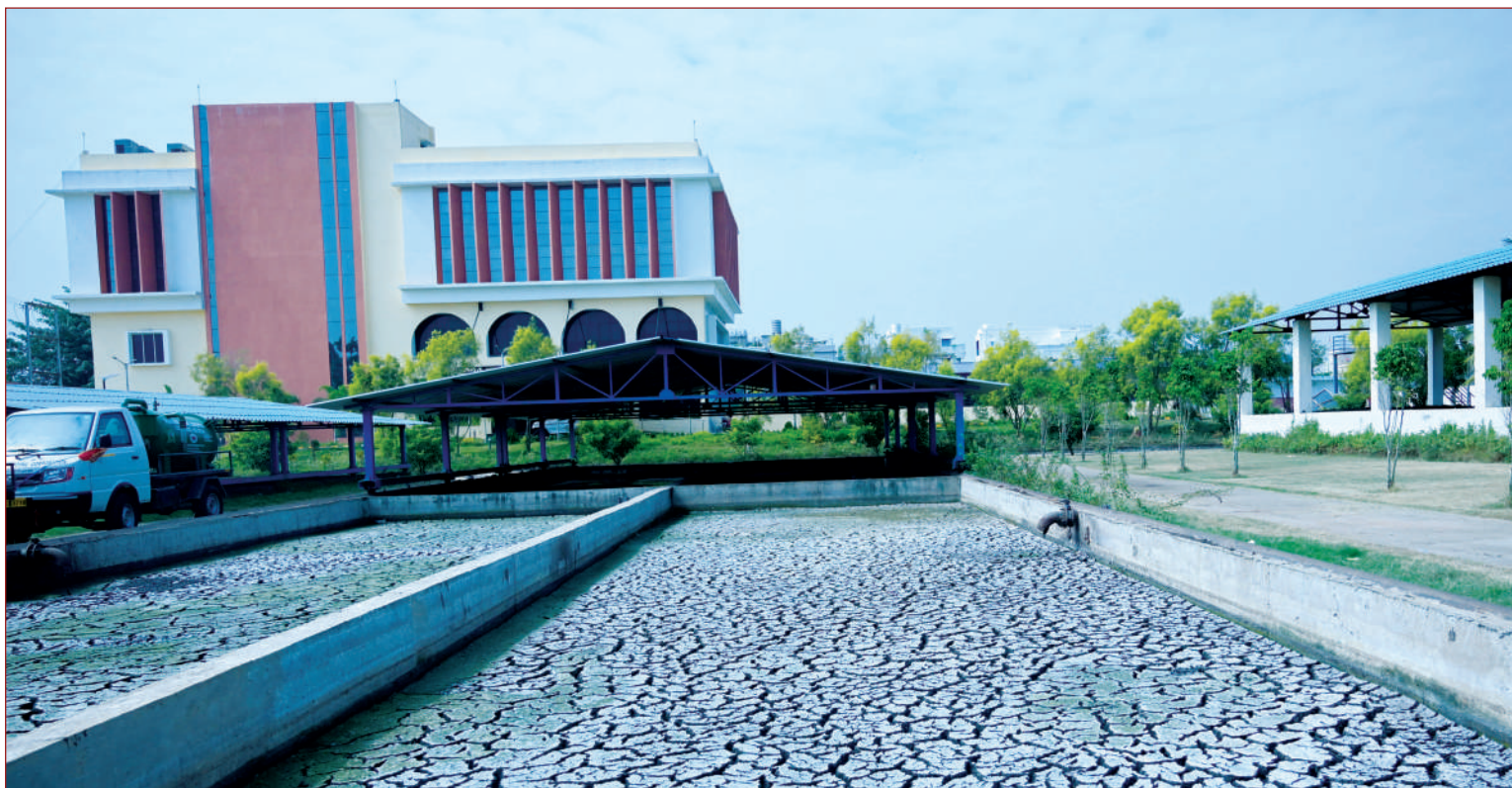
Dry bed of faecal sludge inside a faecal sludge treatment plant (FSTP) in Bhubaneswar, Khordha district, Odisha
