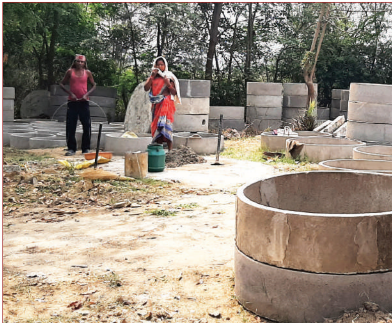
Attempting to meet the growing demand for toilets, masons are diligently engaged in preparing additional rings for septic tanks in Sambalpur, Odisha
