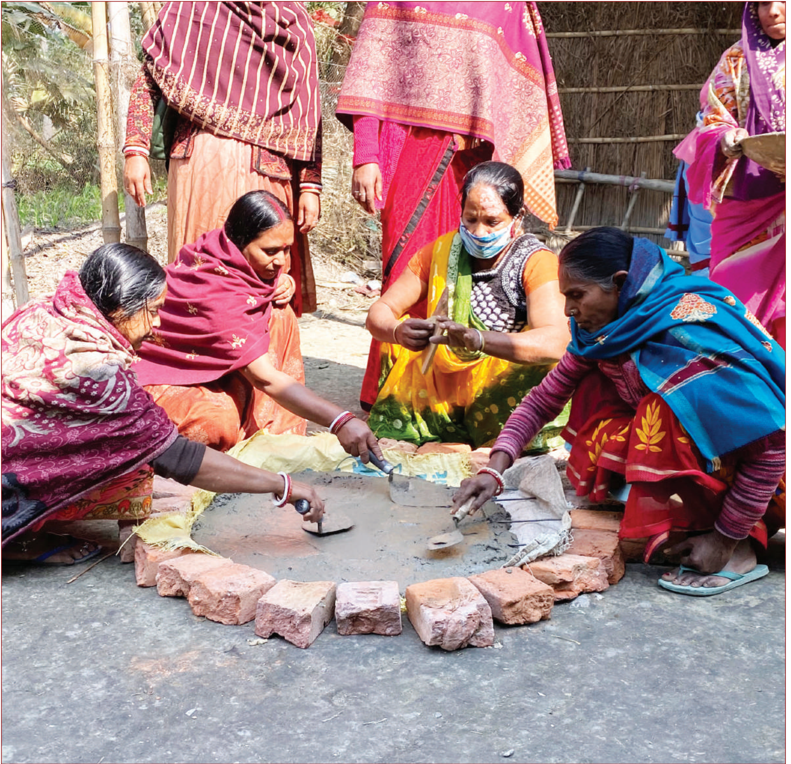
Hands-on training on toilet construction and retrofitting conducted for women masons in Bihar
