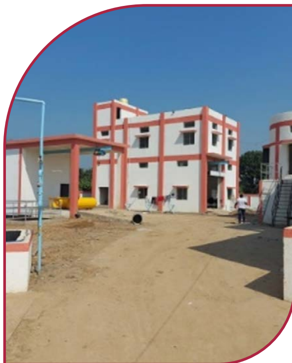
Sewerage Treatment Plant with SBR (Sequencing Batch Reactor) technology of 2.2 MLD capacity
