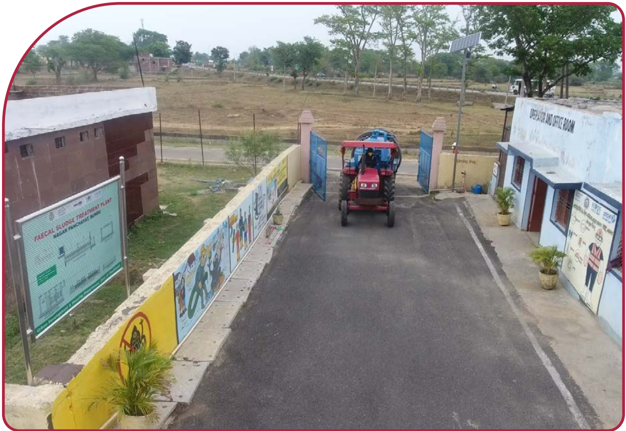
Sludge collecting vehicle entering the FSTP
