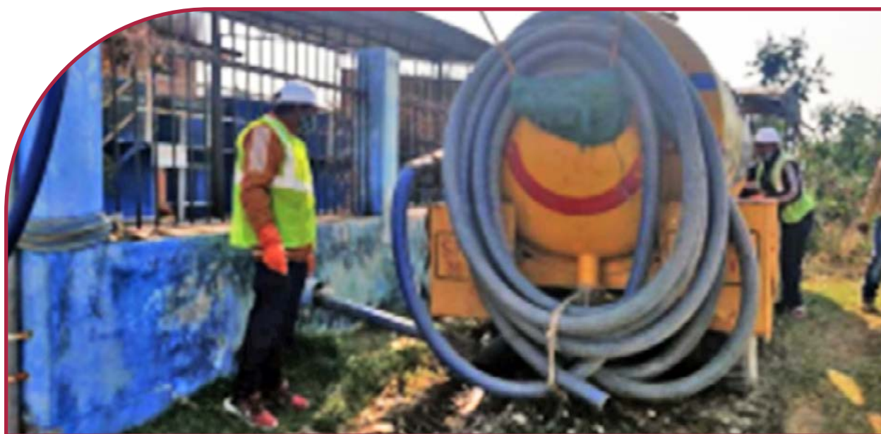
Emptying of Faecal Sludge at the Ambikapur FSTP.
