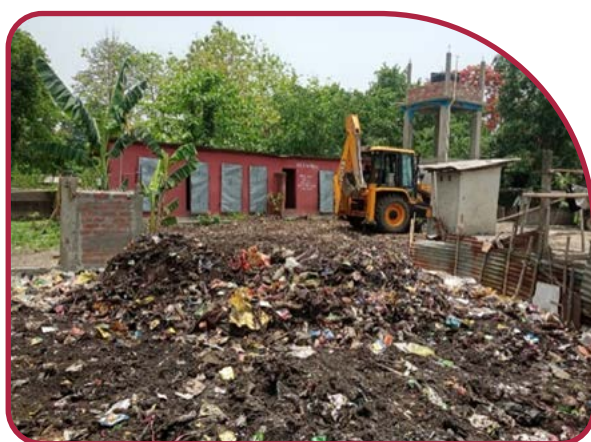
Garbage site being cleared
