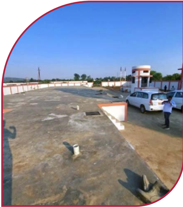
1.2 MLD DEWATS treatment facility at Budhni is servicing approximately 1,000 HHs
