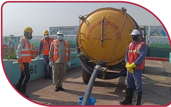
Sludge Collecting Vehicle at the FSTP, Kumhari, Chhattisgarh.
