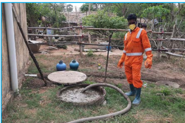
Desludging of single pit in progress in Angul, Odisha
