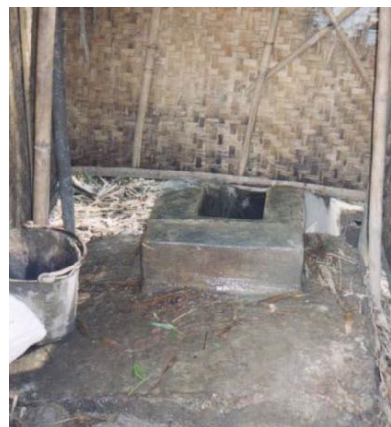
Two vertical bamboo poles can be used for stability when squatting and for assistance when moving from standing to squatting position
