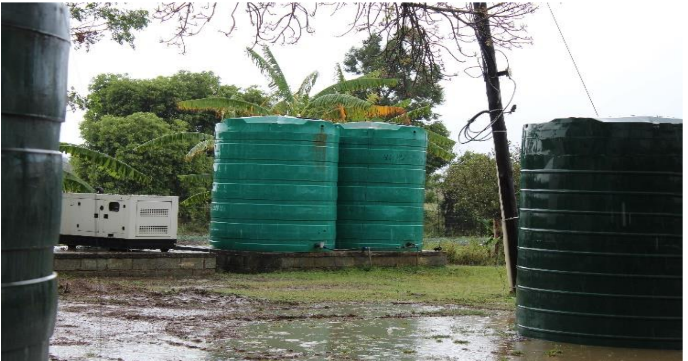
Figure 4: 5000L tanks found in one of the HCFs
