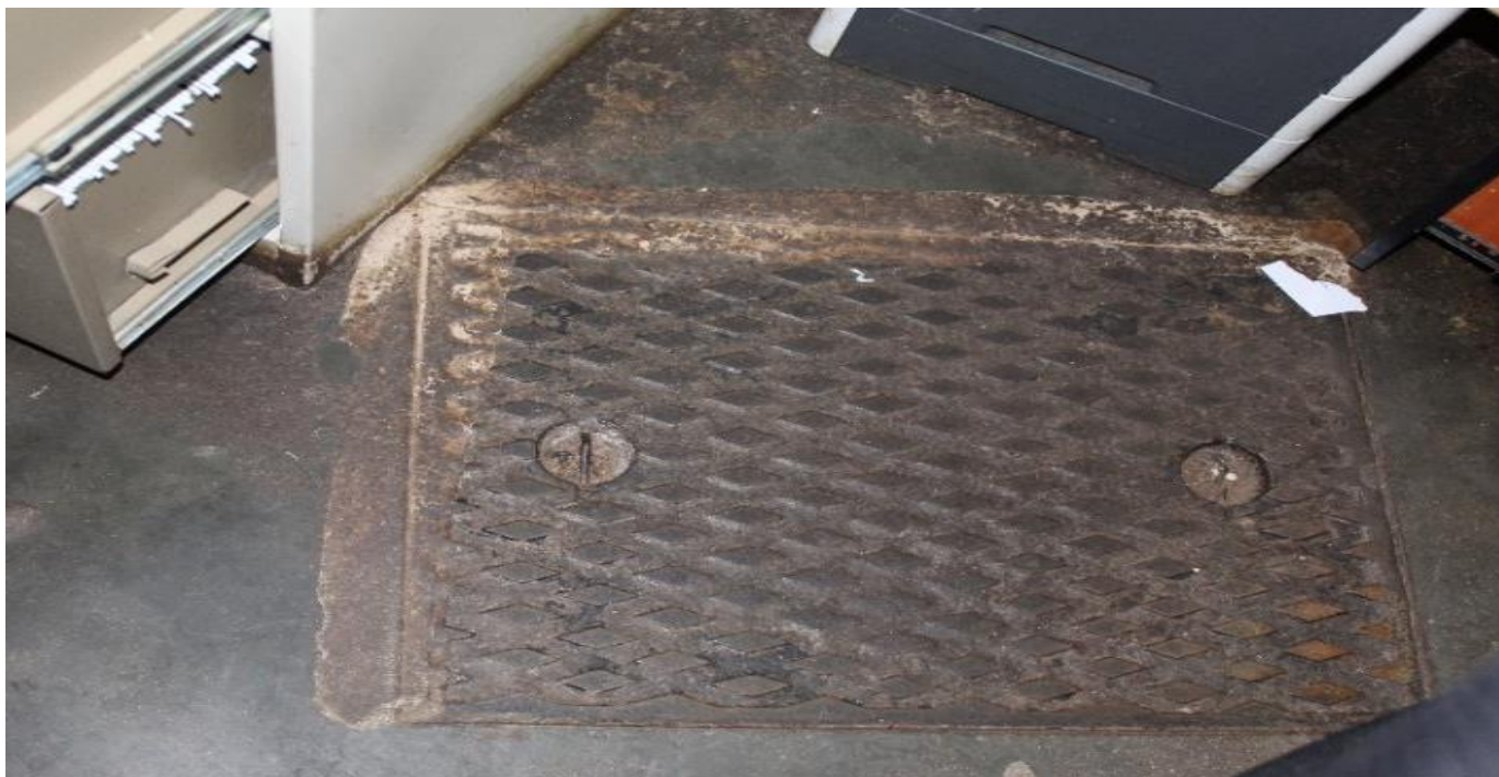
Figure 7: Manhole observed inside a consultation room
