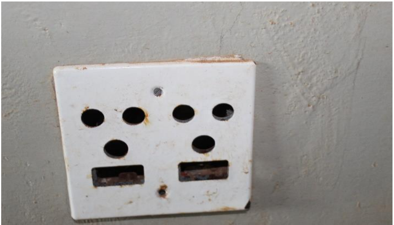
Figure 23: A non-functional plug observed in one of the HCFs
