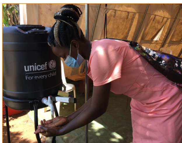
Figure 4: A handwashing facility adapted locally for hands-free usage
