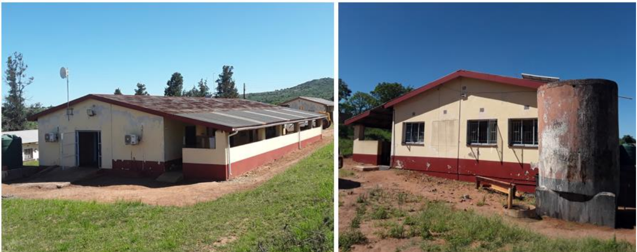
Figure 1: Pictures of Ntjanini Clinic Main Building in Shiselweni Region
