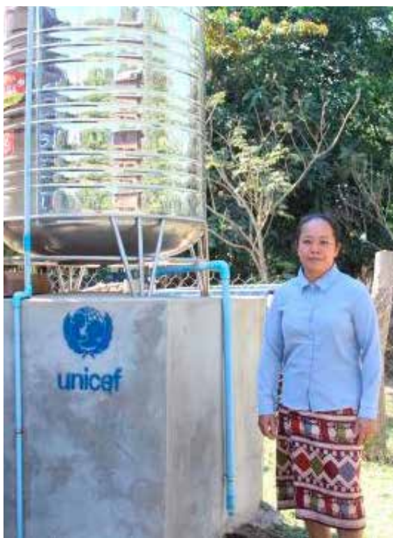
Deputy village chief Naduangchanh shows the new water towers constructed by UNICEF
