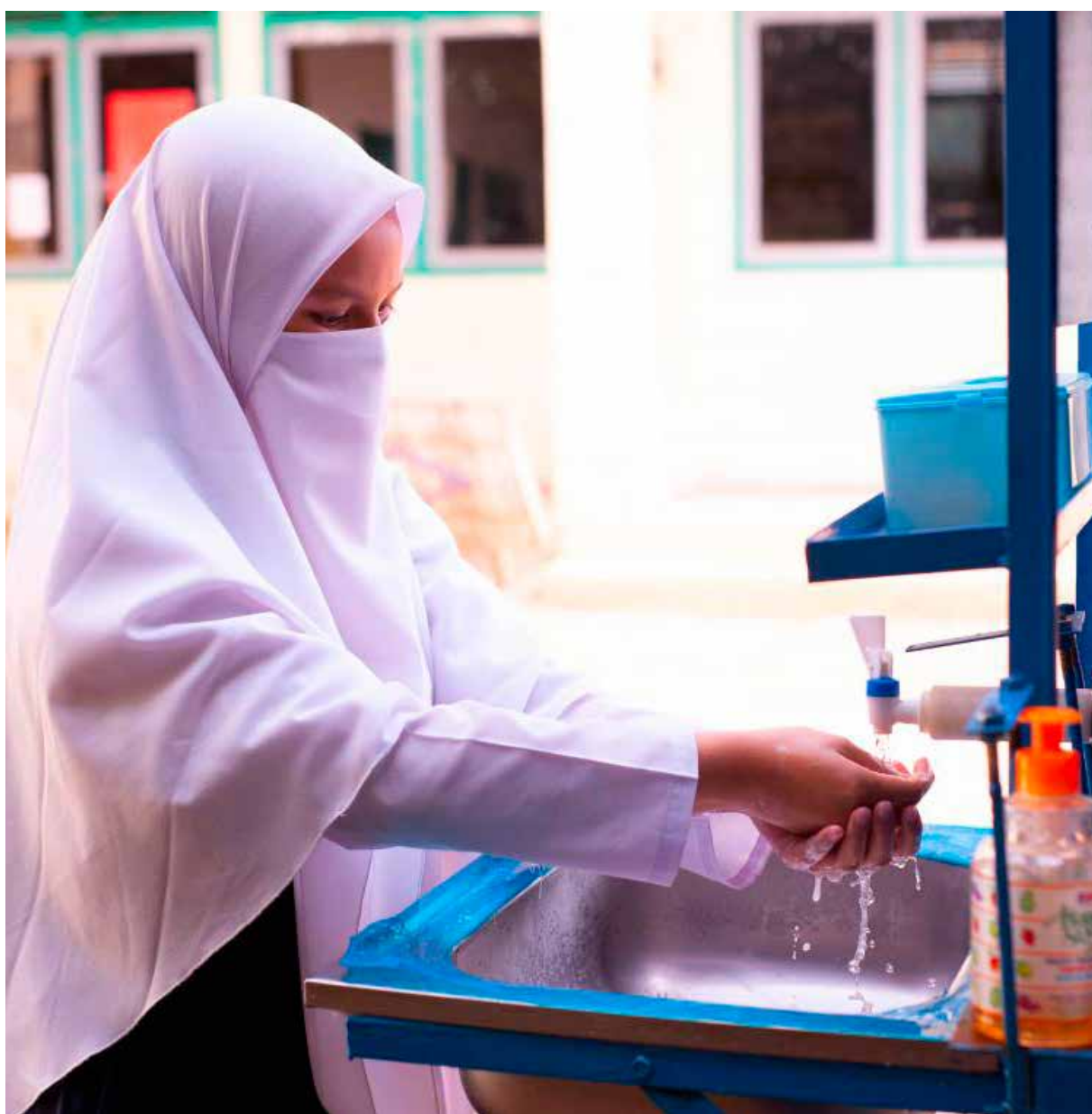
A student washes her hands at a newly installed handwashing facility at her elementary school in Aceh Province © UNICEF/2021/Ihsane
