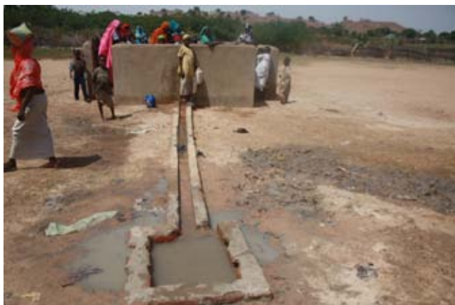
Operational drinking water well with manual pump at Tamassi
