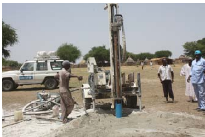
Positive Borehole at the Goza site
