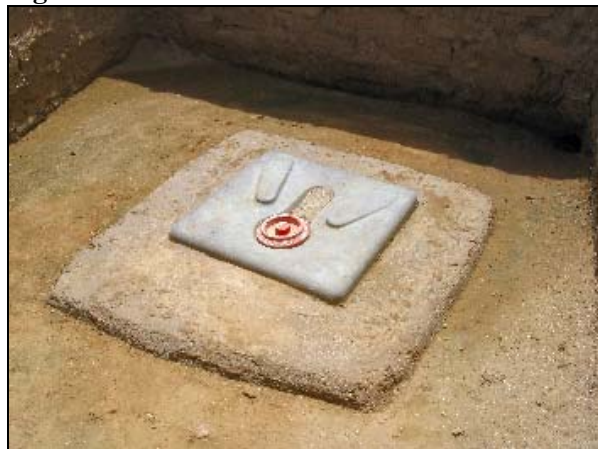
Figure 2: Installed latrine slab
