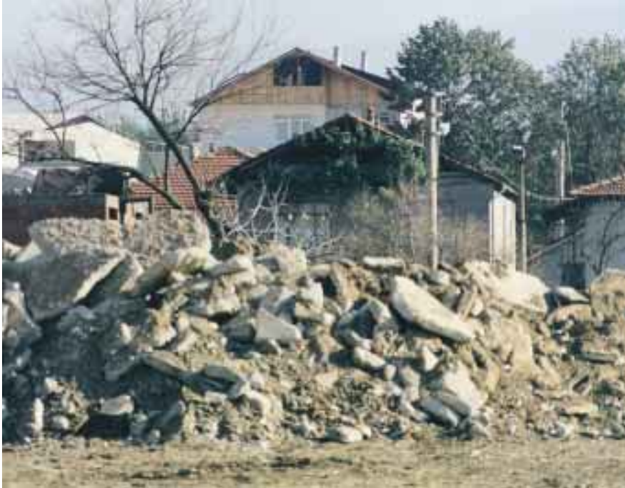
Left: the remains of a ruined street in Gölcük
