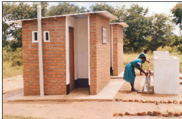
New school latrines and hand-washing stations constructed with UNICEF support, Dowa district
