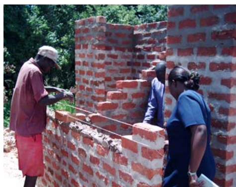
Construction of double pit latrine under DAPP Namwala
