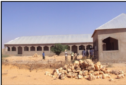
Wisil School under construction © UNICEF Somalia/2011
