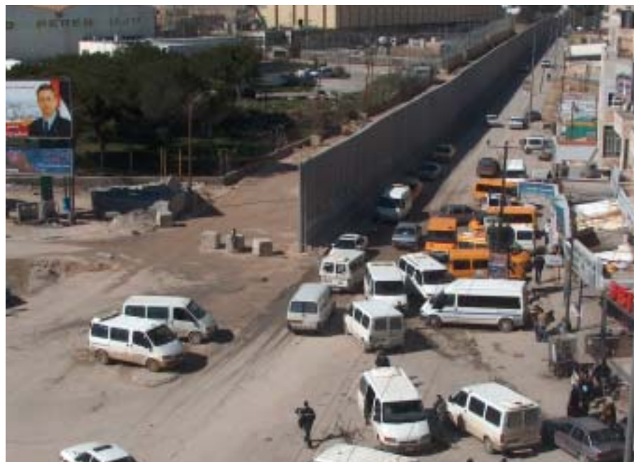
The Barrier under construction down the middle of the road in Ar Ram.
