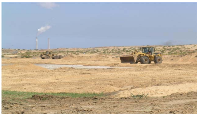
Emergency repairs being carried out to backfill the damaged embankment © UNICEF
