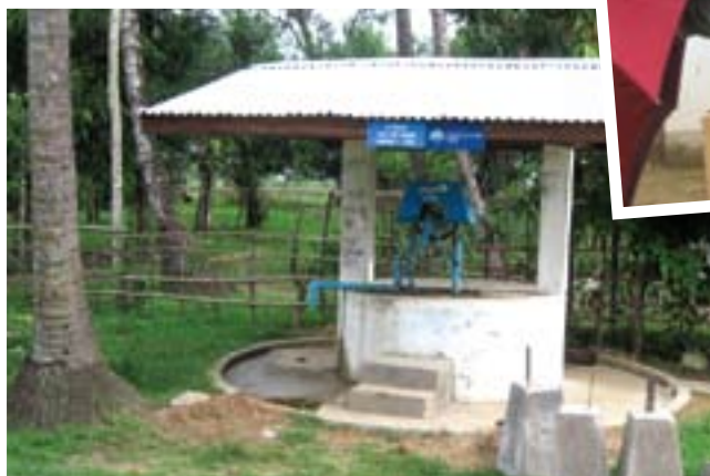
This rope pump was established after the NRS floods as a safe water source in Buthidaung Township
