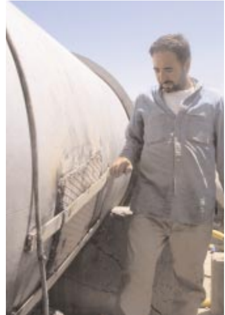
The pipeline after UNICEF repairs
