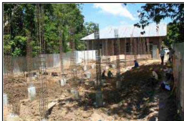
Construction is underway in the village of Ulee Tuy.
