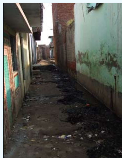
One of the streets in Abbas Nagar before the Urban Sanitation and Hygiene Action (USHA)
